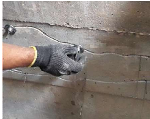
Figure 6.4: Attaching the adhesion nozzles
