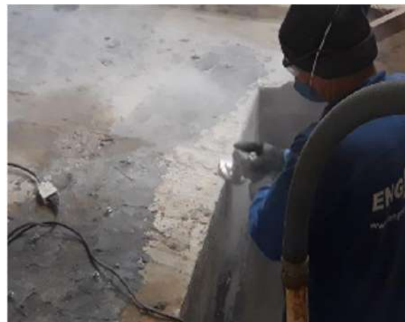
Figure 8.2: Regularization of block surfaces and corners using a sander
