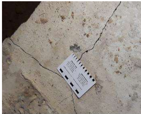
Figure 5.3: Crack measurements performed by fissurometer
