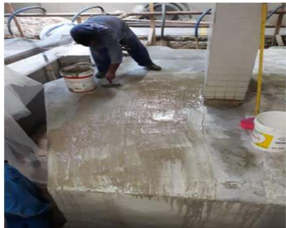
Figure 8.4: Application of waterproofing product
