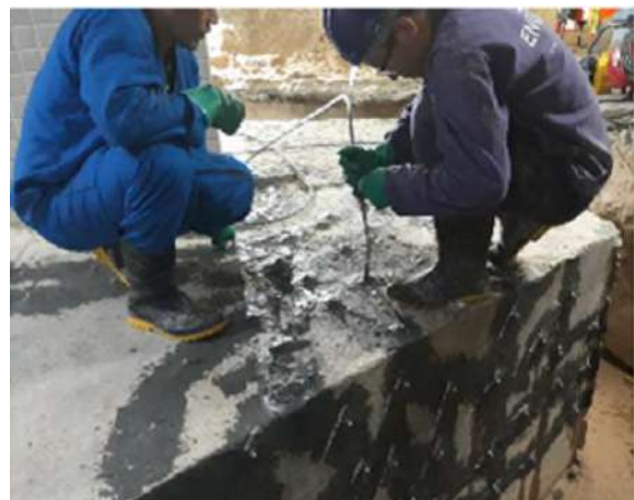
Figure 7.2: Injection of epoxy resin into the foundation block
