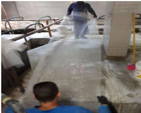
Figure 8.5: Screen being applied to the block
