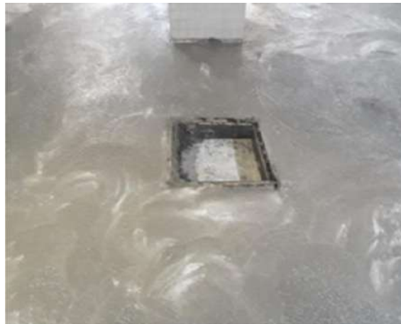
Figure 9.1: Construction of the floor and inspection window
