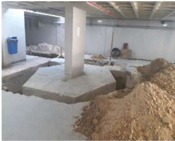
Figure 5.1: Exposed foundation block
