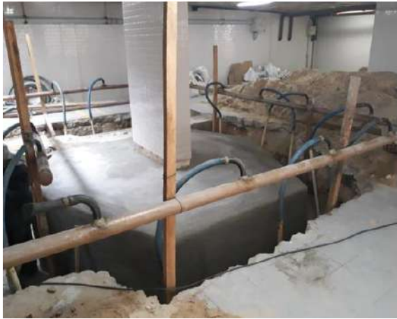
Figure 8.3: Groundwater lowering system
