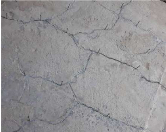
Figure 6.1: Open cracks
