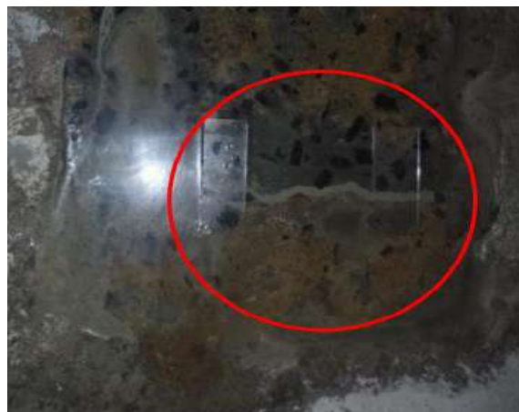
Figure 9.3: Detail of the sealed crack
