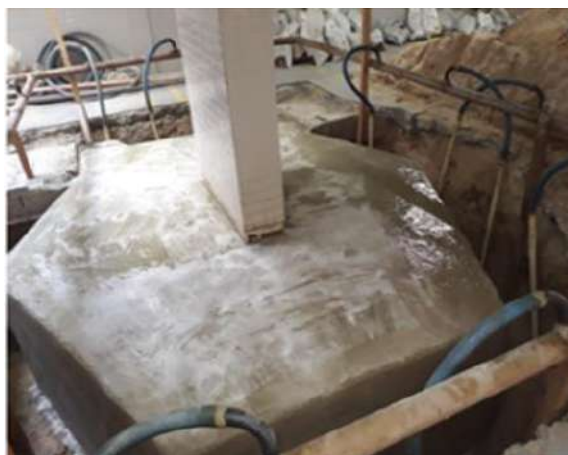
Figure 8.7: Block after waterproofing
