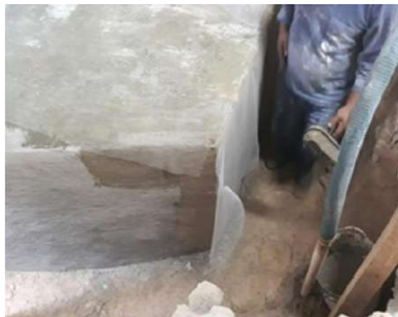
Figure 8.6: Screen being applied to the block corners
