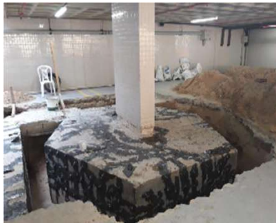
Figure 7.3: Foundation block with cracks filled with epoxy resin
