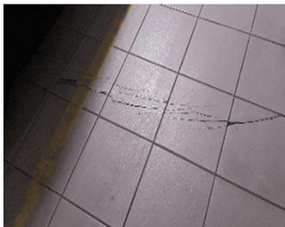
Figure 3.1: Cracks on the floor
