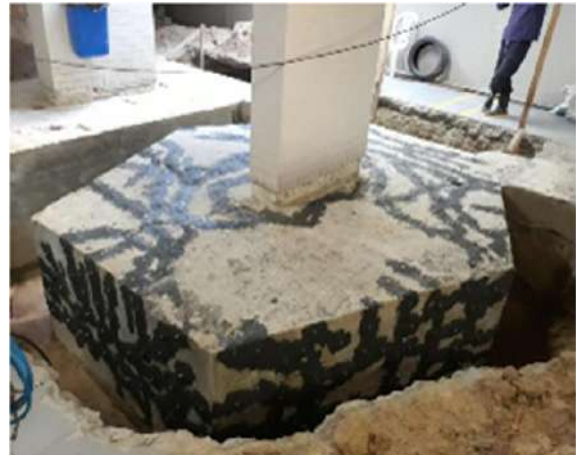
Figure 6.6: Block following crack sealing
