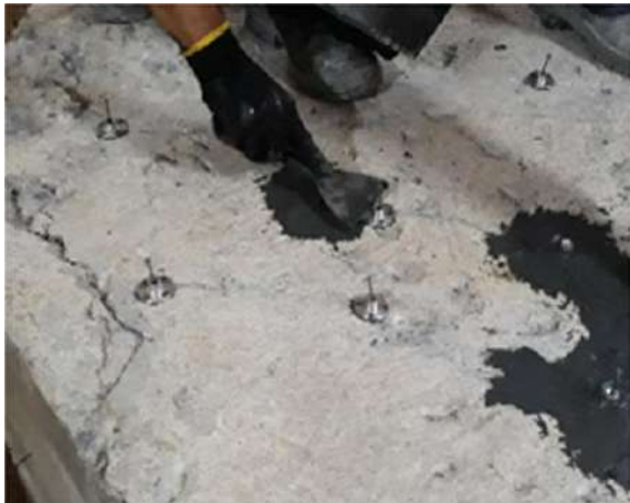
Figure 6.5: Application of structural adhesive to cracks
