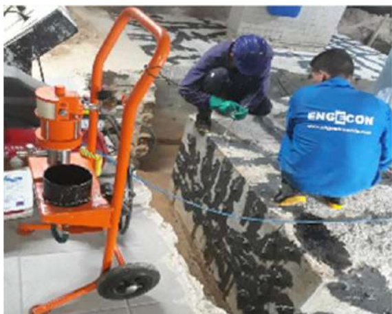
Figure 7.1: Use of Injection pump to apply epoxy resin
