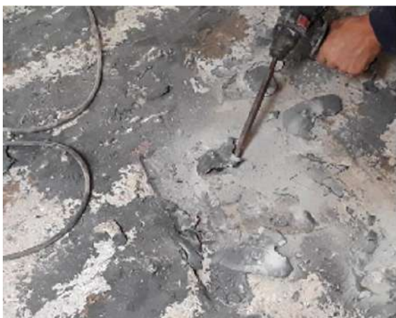
Figure 8.1: Removing the adhesion nozzles
